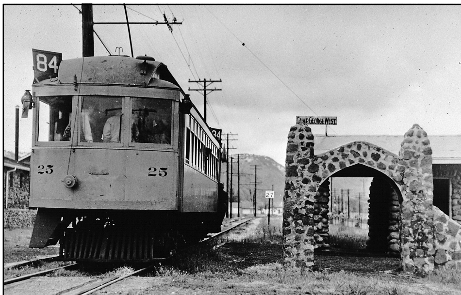
D&IM No. 25 on a Rocky Mountain Railroad Club trip stopped for photos at the Camp George West National Guard Camp Trolley stop before heading into Golden. – May 18, 1952, photo © Richard Kindig.
