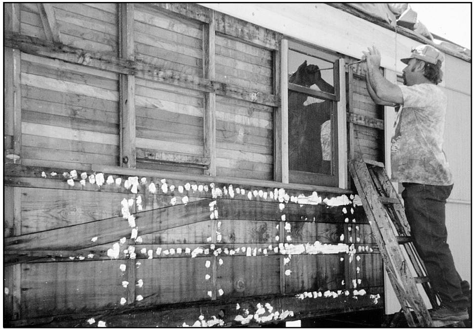
Denny Haefele is installing new hardwood window framing and a sash. The photo shows the new letter board and the new siding to the right as well as the extensive side framing. The spots on the lower portion indicate old nail holes that have been filled.
